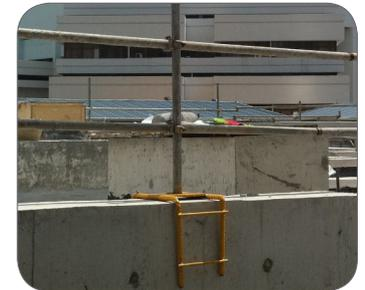
Figure 31: Example of parapet edge protection design.
