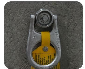
Figure 2: Example of a cast-in eyebolt anchor.
