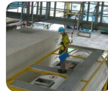
Figure 36: Drive-in anchorage and lifeline structural system.
