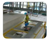
Figure 36: Drive-in anchorage and lifeline structural system.
