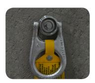
Figure 2: Example of a cast-in eyebolt anchor.
